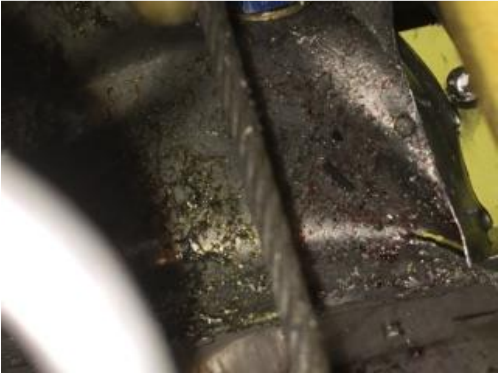
Photo 4 – Structural Damage (FAA Photo)
