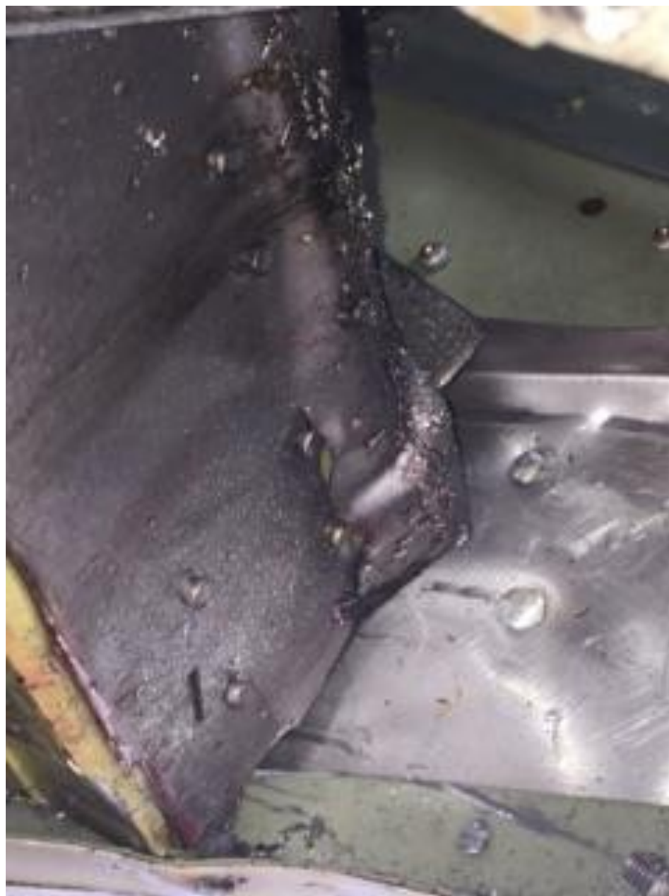
Photo 5 – Structural Damage (FAA Photo)
