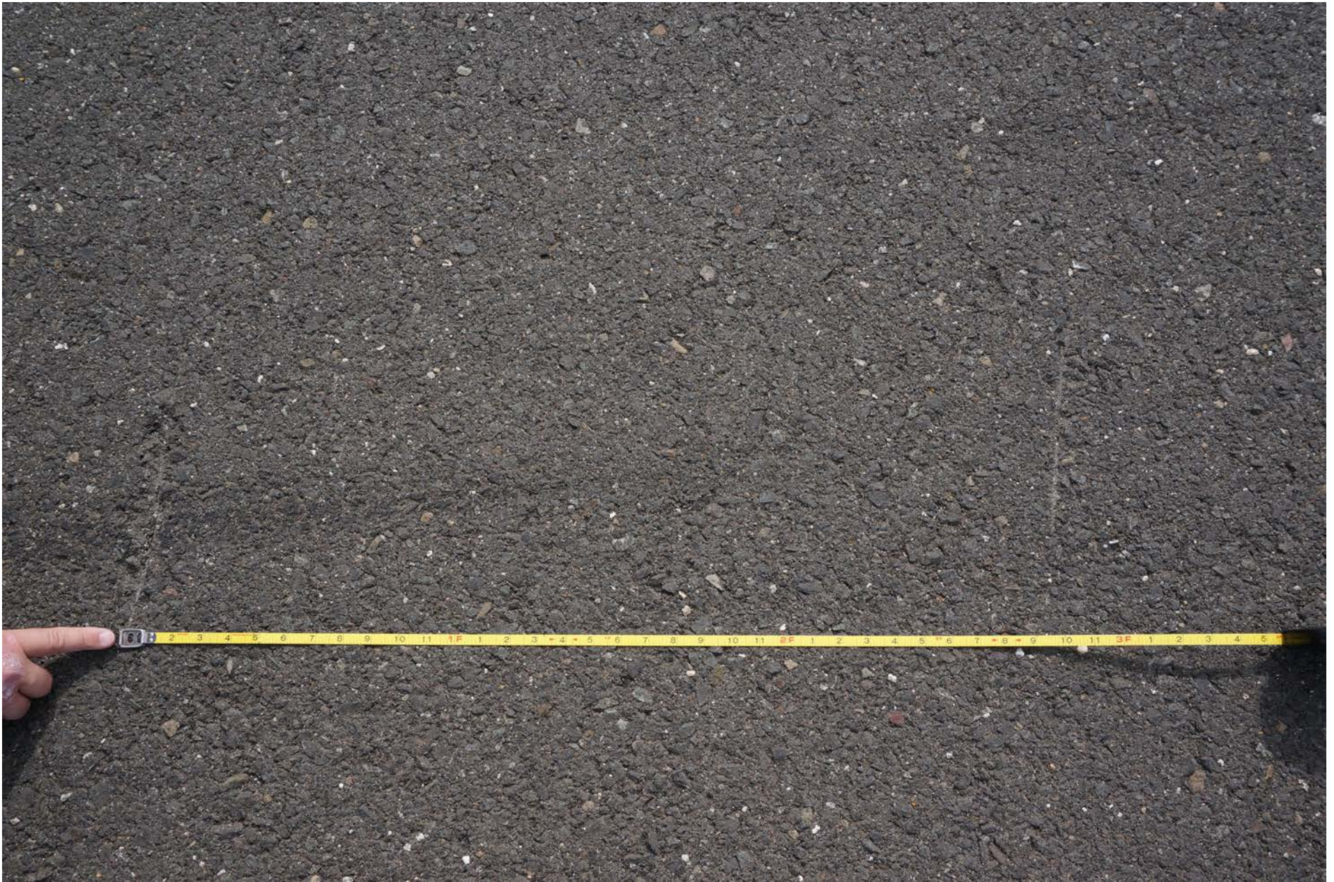
Photo 17 – Close Up of Propeller Strike Marks on Runway
