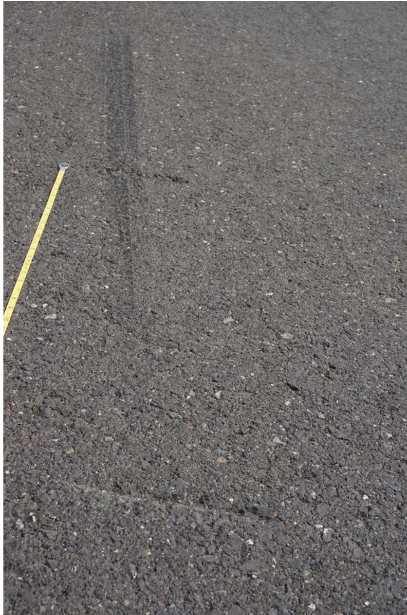
Photo 18 – Tire and Propeller Strike Marks on Runway
