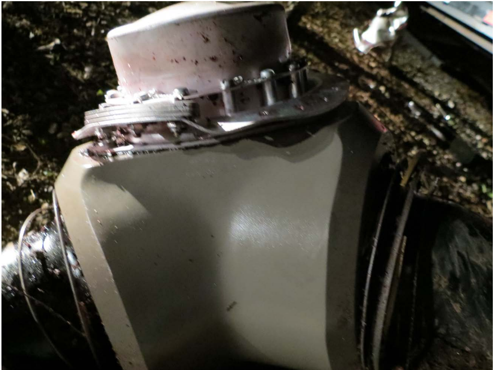
Photo 19 - View of damaged propeller hub
