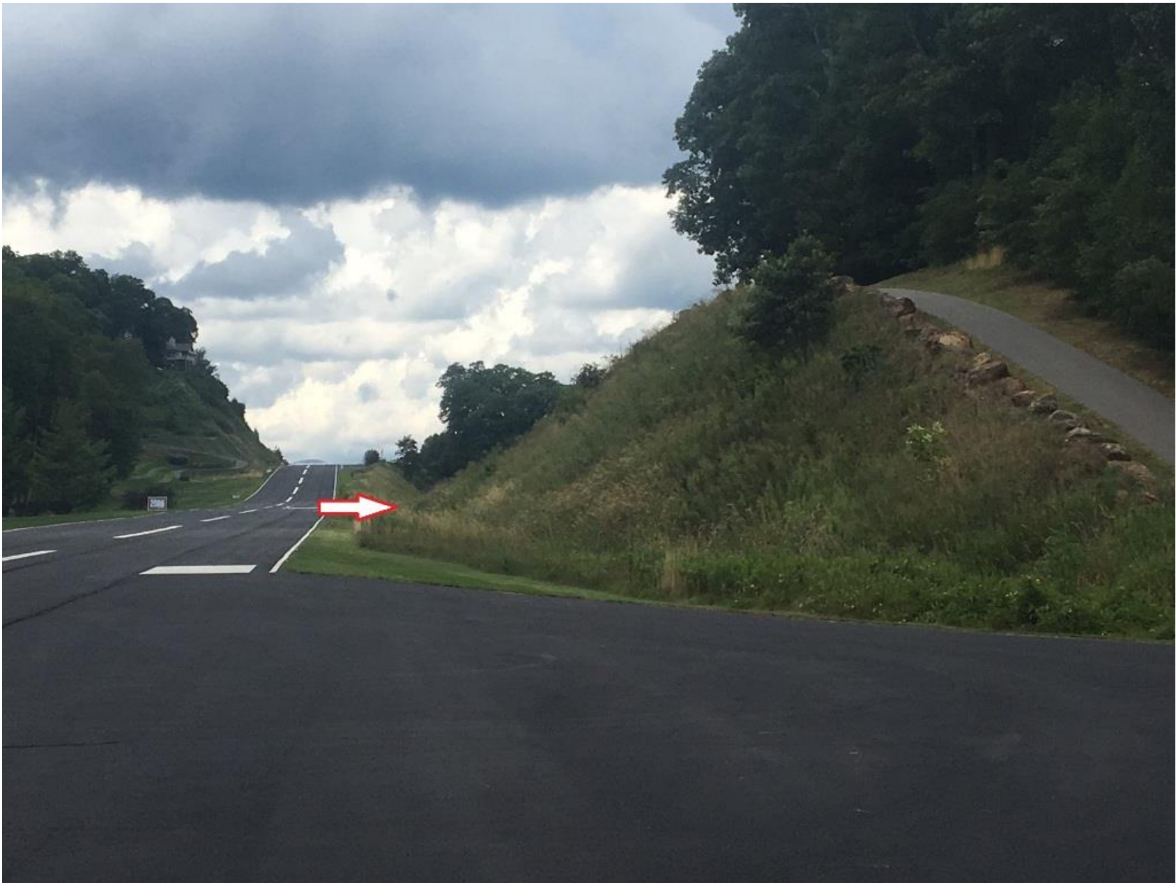
Photo 1 – FAA Digital Photograph. Arrow Depicts the Reported Location of the Bush that the Right Wing Contacted
