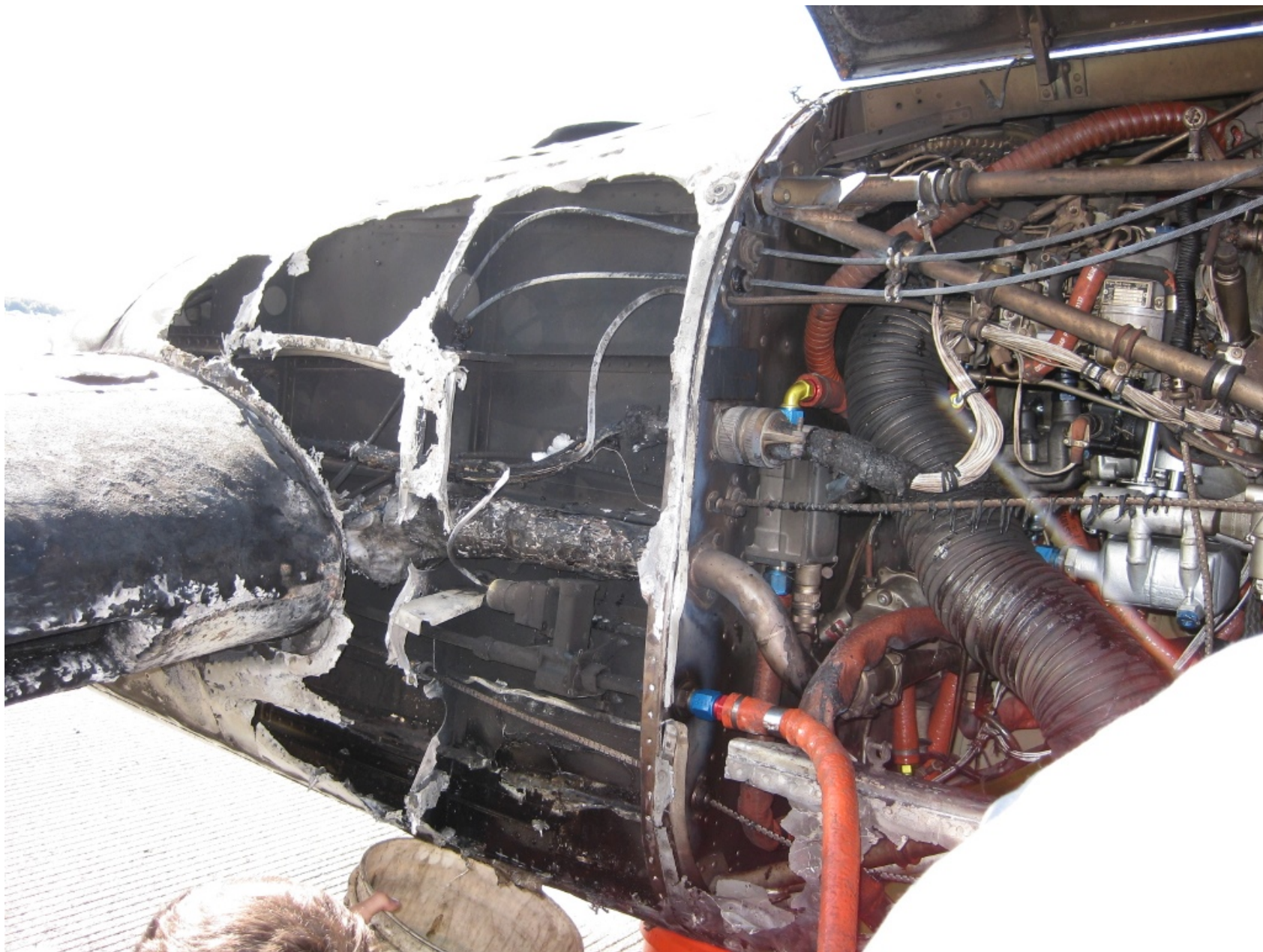
Photo 3 – View of fire damage to left engine nacelle (Provided by FAA)
