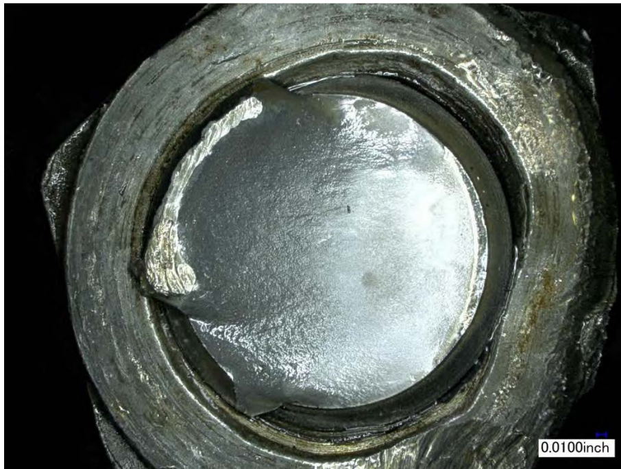
Figure 9 Bolt fracture surface
