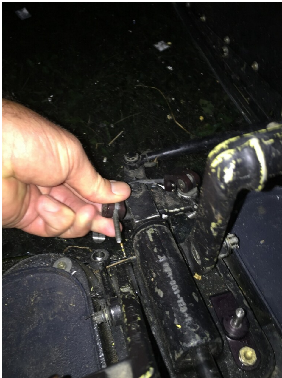
Photo 3 – View of Fractured Pin (Operator)
