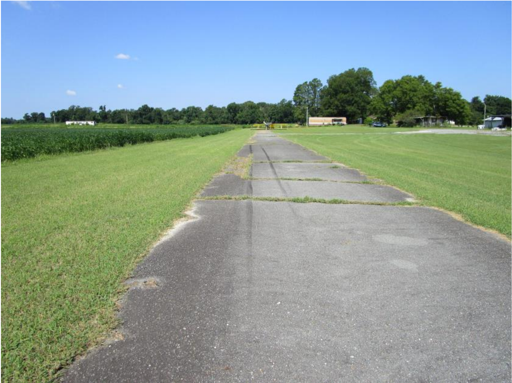
Photo 5 – Airplane at Rest from Approach End of Paved Surface (Courtesy of the FAA)
