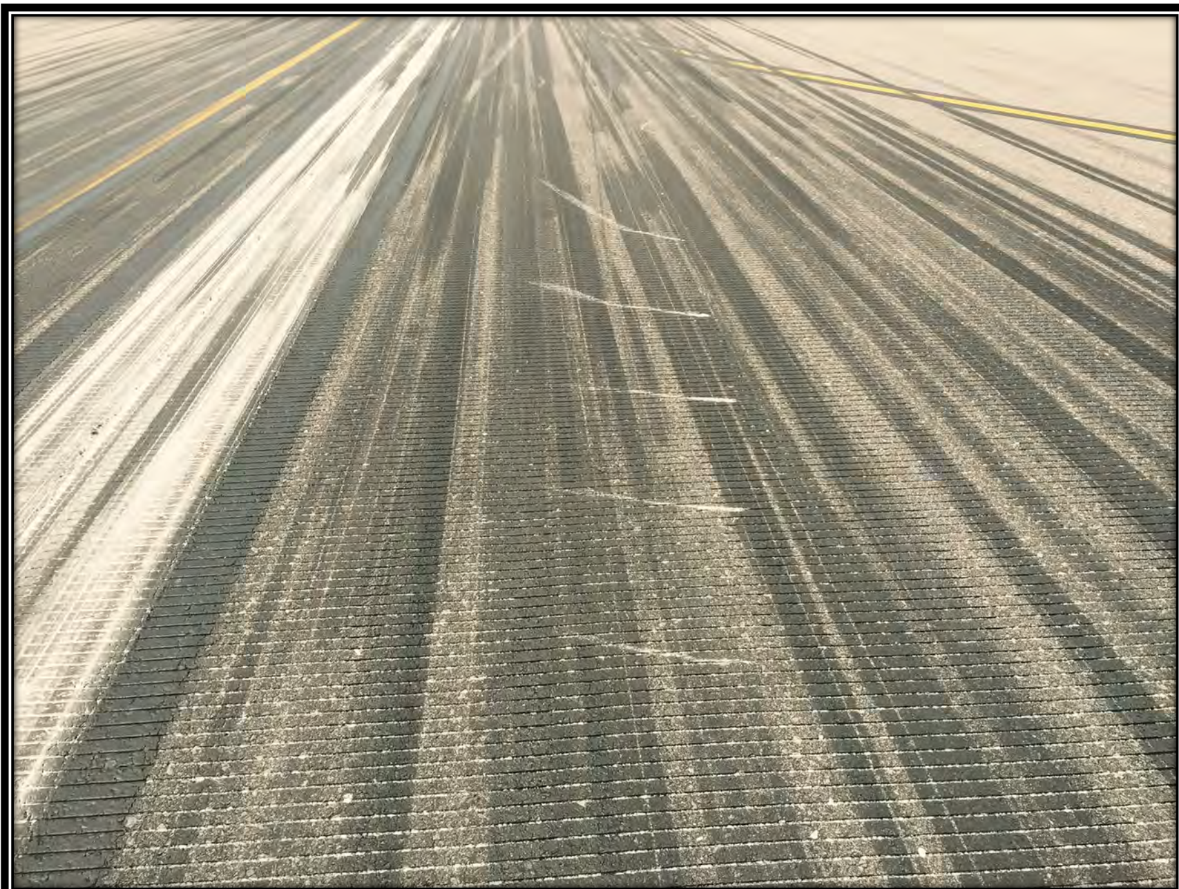
Photo 2 – Close Up View of Runway Scars (Photo Courtesy of FAA)
