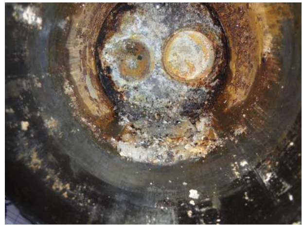
Photo 34: Cylinder No. 3 Barrel after Removal
