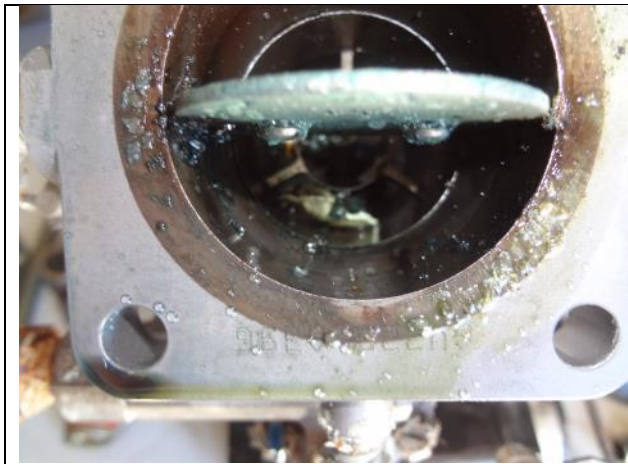
Photo 37: Carburetor Valve as Found
