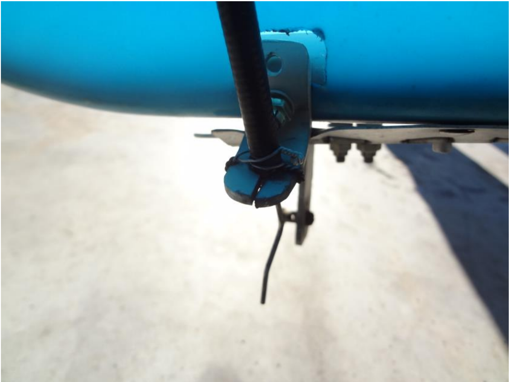
Photo 7 - Elevator Cable and Clamp as Viewed
