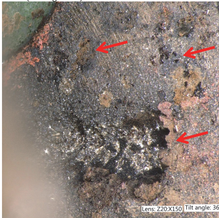
Figure 20. Blackened surface of the switch module header, with visible pitting (upper arrows), undercutting, and flaking (lower arrow). This surface was beneath one of the terminals where a wire had been attached.
