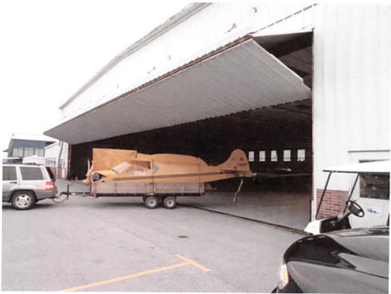
15. Hangar 2, Lock Haven William T. Piper Memorial Airport
