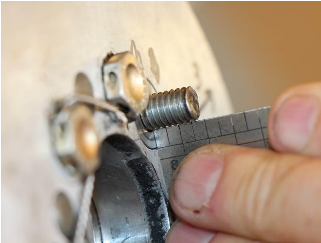
Photo 10 - Measurement was 0.46 inches at bolt (B).
