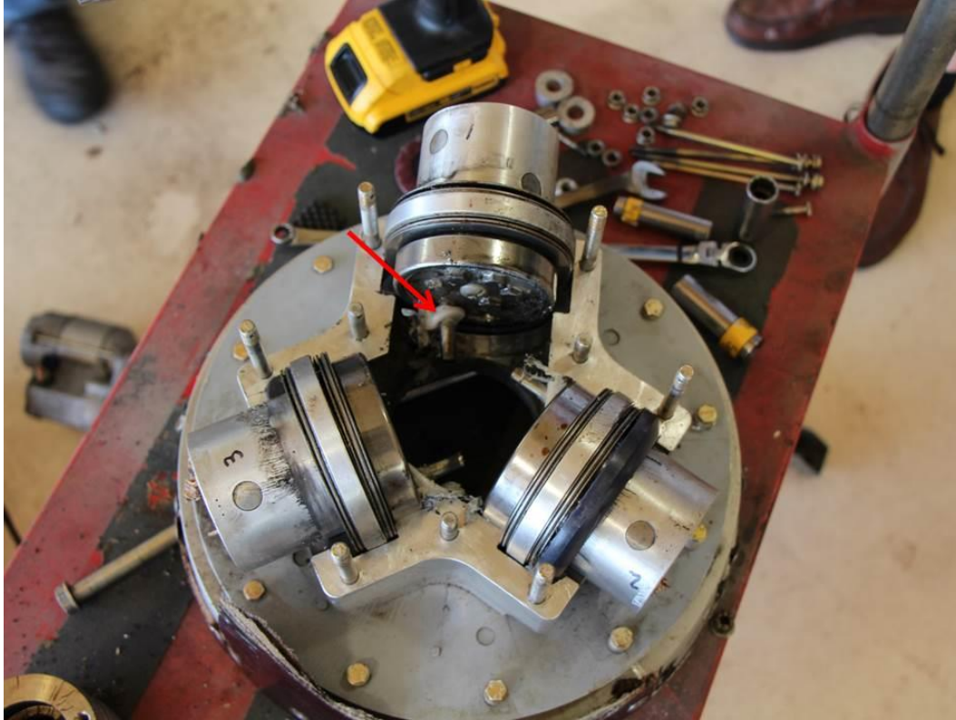
Photo 22 - The arrow points to one of the melted Delrin bushings. The Delrin bushings fit over the blade's pitch change pin. The pin and bushing fit in a groove in the blade pin spool (removed).
