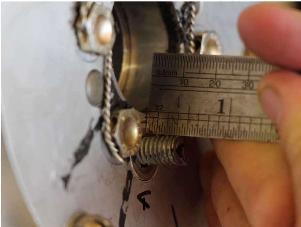
Photo 9 - Measurement was 0.41 inches at bolt (A).
