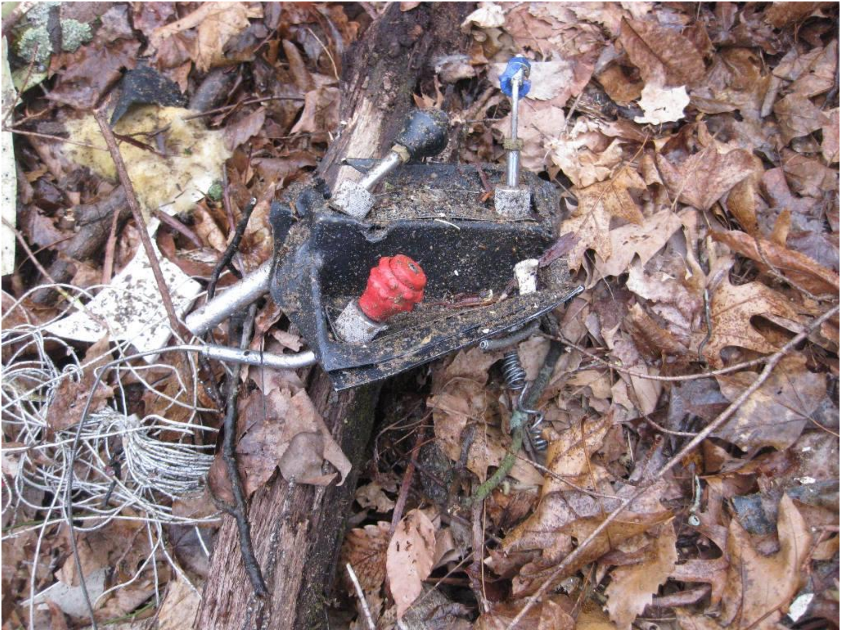
Photo 8 – Engine Power Panel
