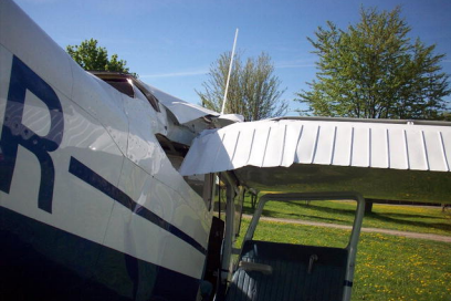
Photograph # 1: Right Wing Damage (Photo Courtesy of [redacted])
