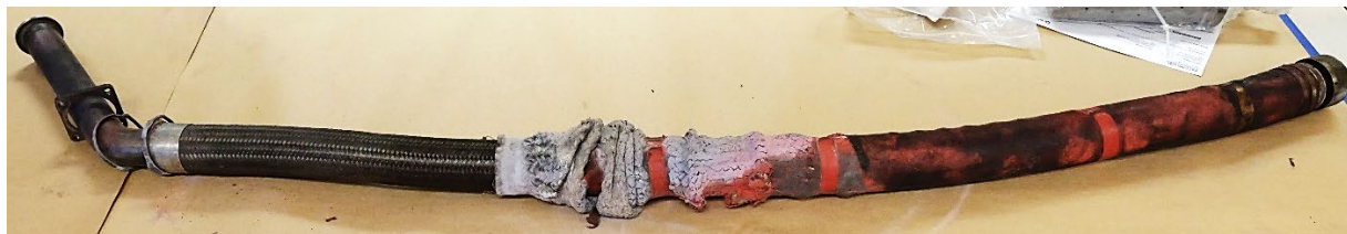
Figure 20: Fire sleeve pulled back
