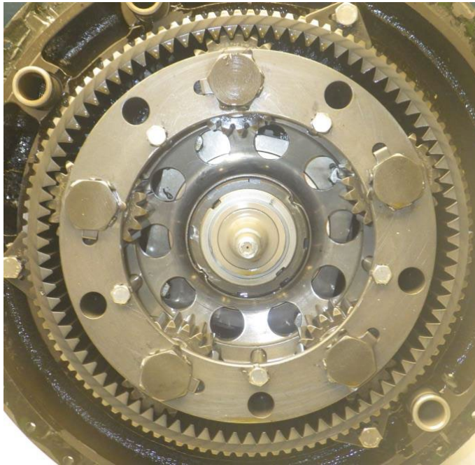
Photo 21 - 2 nd Stage Reduction Gear Assembly - Undamaged
