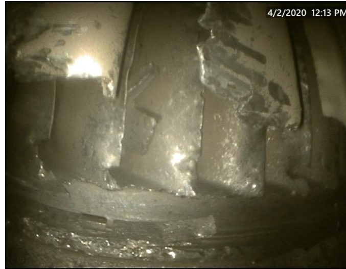
LPT Stages 1-5 showed missing airfoils and nozzle distress
