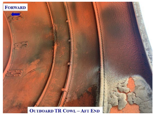
PHOTO 6: RIGHT TR DISTRESS
