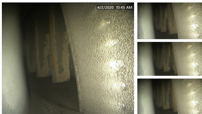
PHOTO 26: NO HPT ROTOR SECTION DAMAGE
