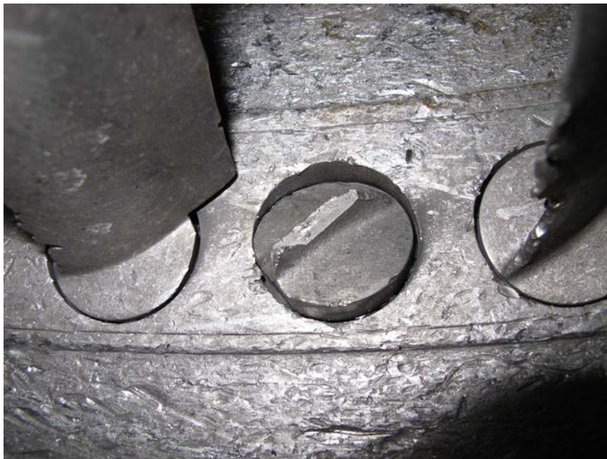
Photo No. 9: View of the fractured outer end of the 5th stage VSV in the lower compressor case half. (P&W)
