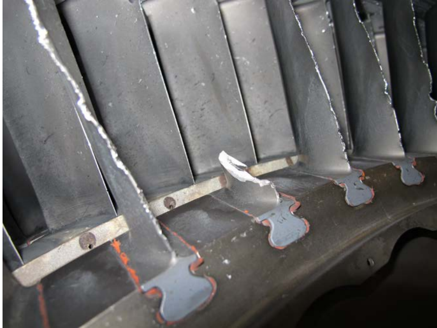
Photo No. 17: Close up view of fractured 4th stage compressor blade. (P&W)
