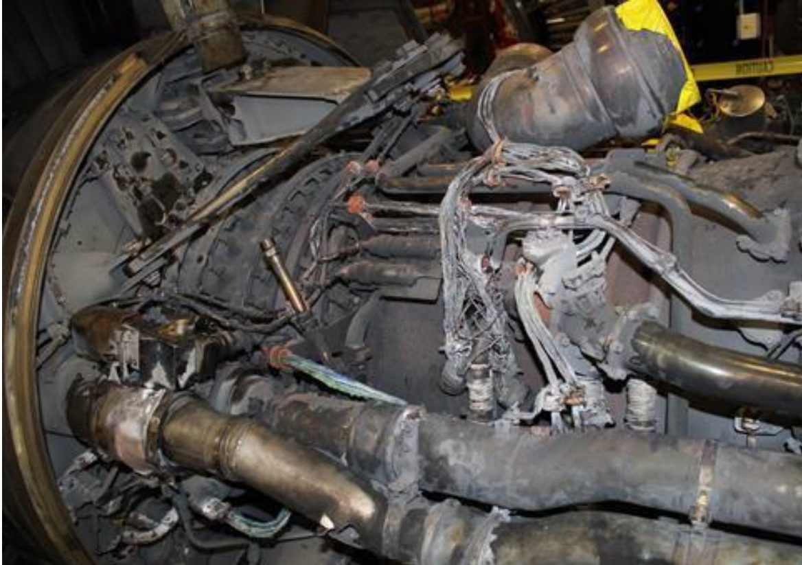
Figure 9. General thermal distress, engine externals on left side of the engine
