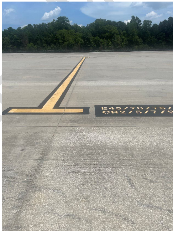
Figure 8 – CHS RON Ramp Spot R6 J-Line/Stop-bar
