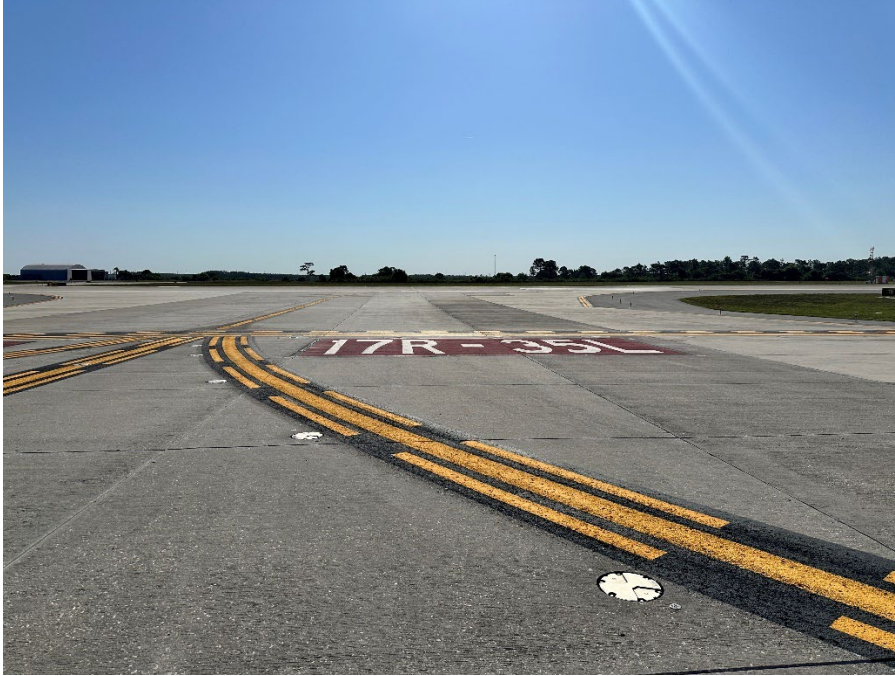
Figure 7: View of Runway 17R/35L Hold-short Line and Taxiway Markings on Taxiway H2 (Source: Human Performance Group Chairman)
