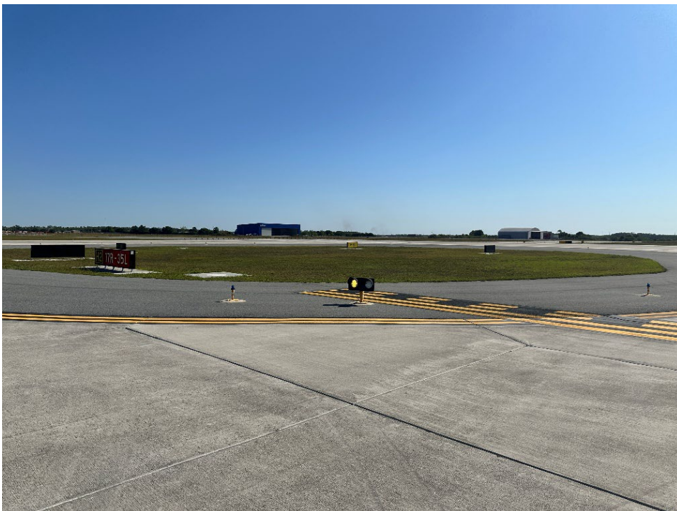
Figure 6: View of Hold-short Line and Runway Sign for Runway 17R/35L (Source: Human Performance Group Chairman)
