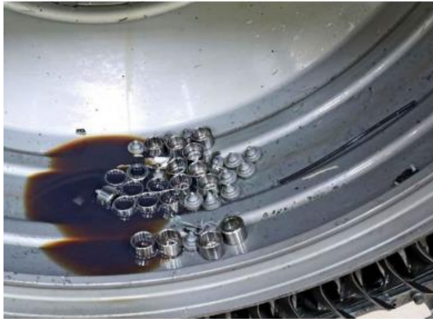
Figure 3: Oil and Sheared No. 1 Bearing Housing Support Bolts in Booster Cavity
