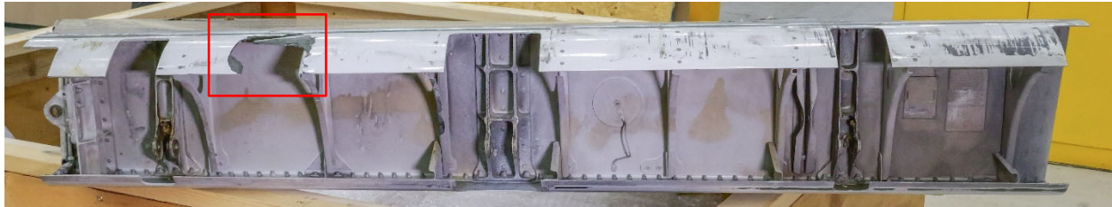
Figure 57: Section of material missing from LH elevator assembly, forward looking aft
