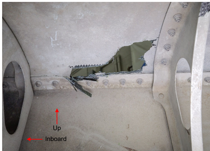
Figure 47: Inner surface of the RH elevator damage
