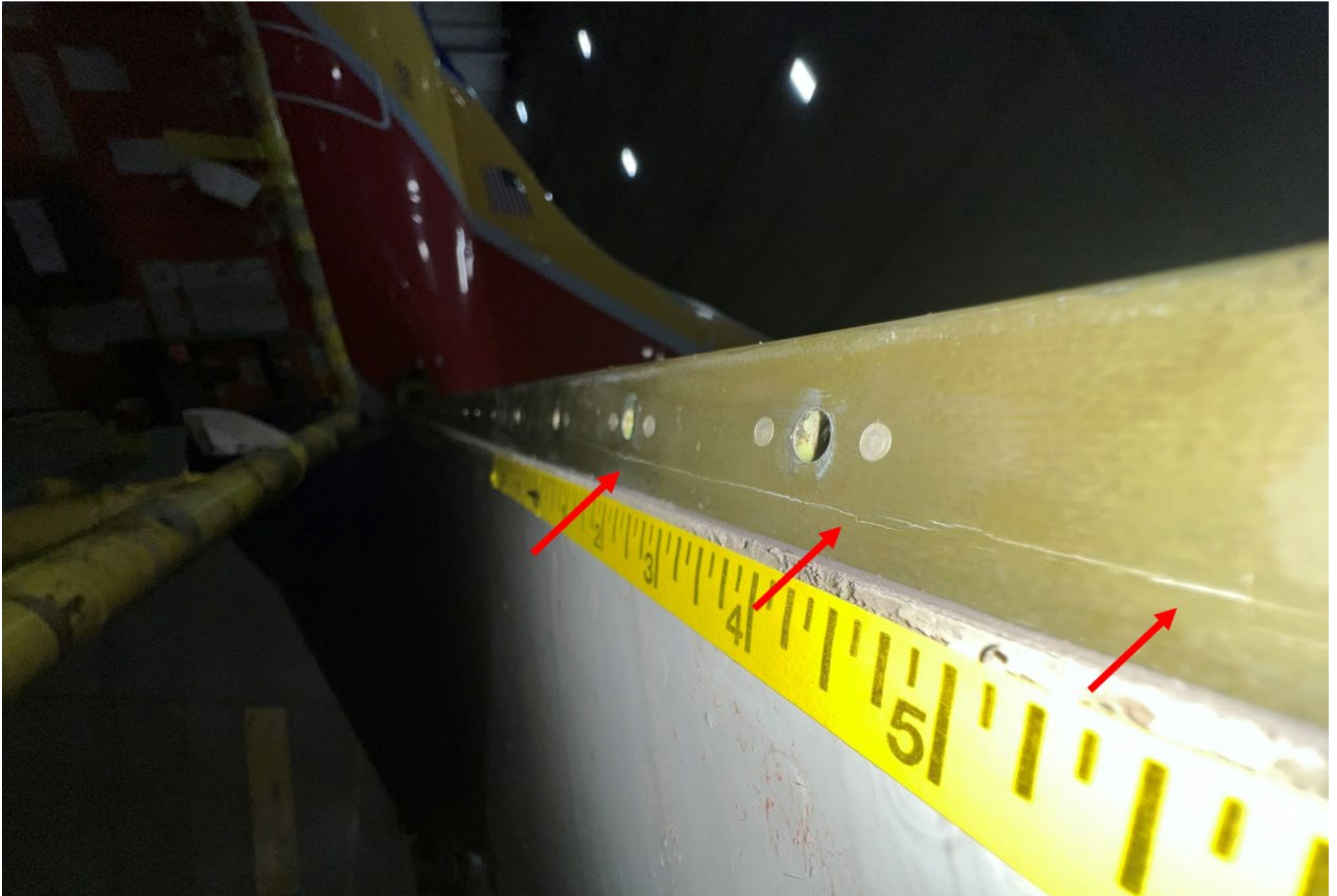
Crack on Bottom face of Lower Spar Chord (courtesy SWA)
