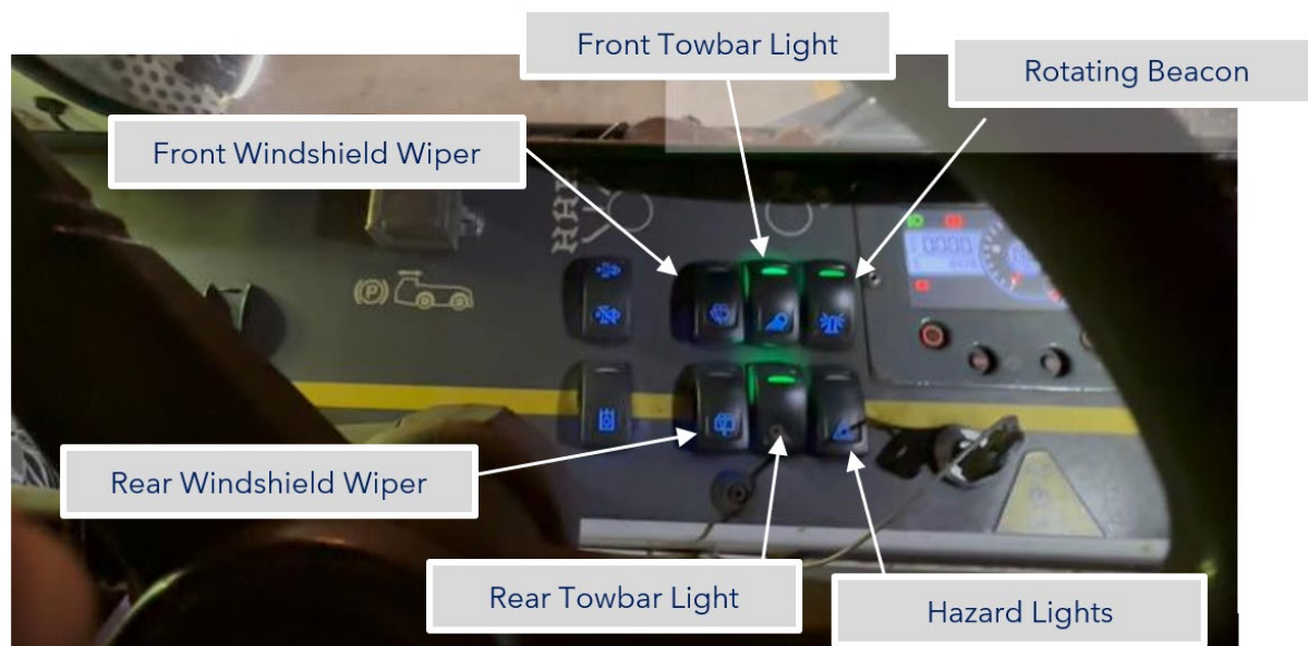
Figure 9: Switch panel on the dashboard of the tow tractor. In this photo, the front tow pin spotlight, rear tow pin spotlight, and rotating beacon are selected on.
