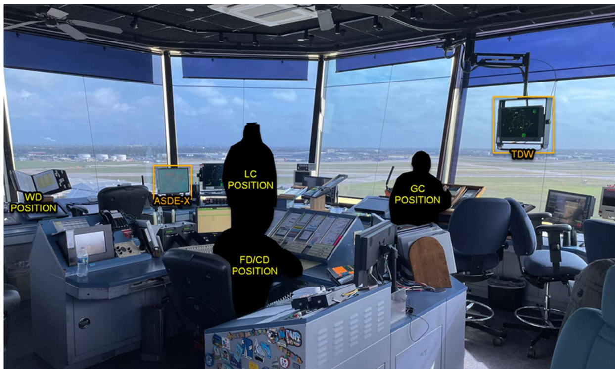
Figure 5. Tower cab with controller and pertinent equipment locations.
