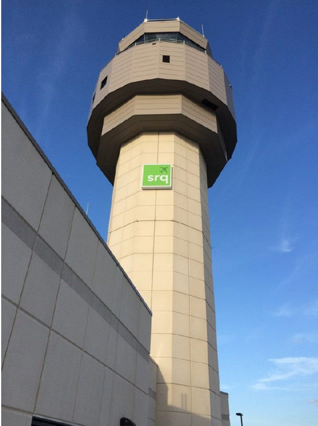
Figure 5. Photo of SRQ ATCT. Photo credit: Unknown.
