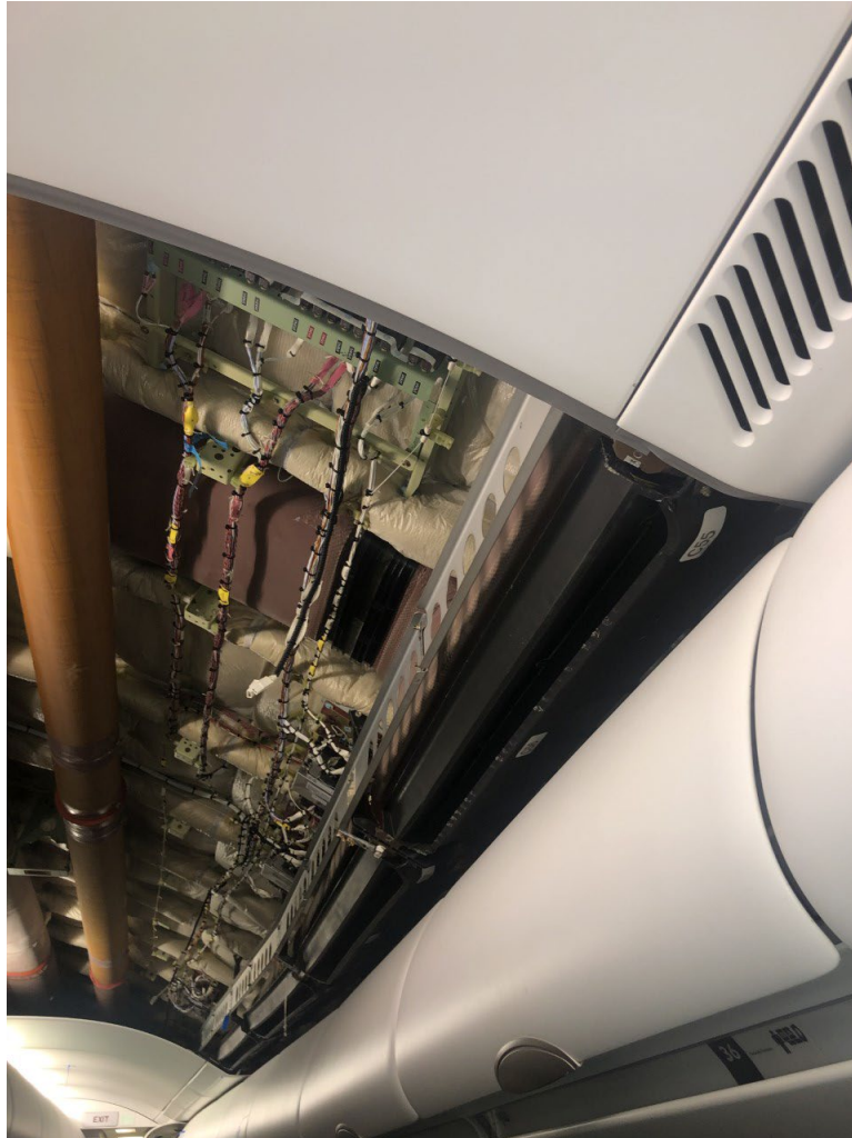
Figure 3. Missing ceiling panels near rows 36 through 41.
