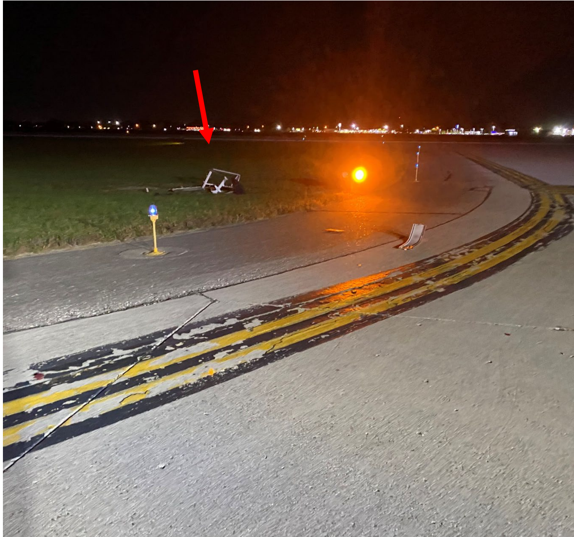
Photograph 4 - View of Damaged Sign (Courtesy Air Wisconsin)
