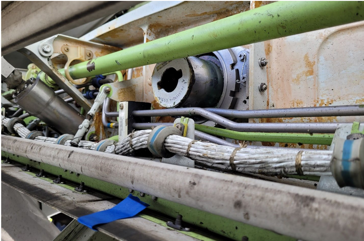
Figure 5. View of the opposite end of the forward remnant of the aft trunnion pin shown in Figure 3.
