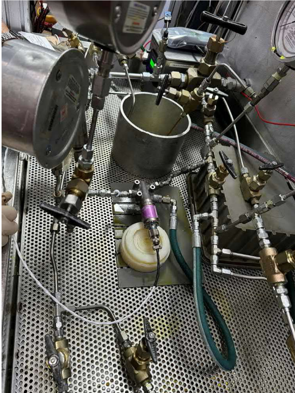
View of the part while plumbed on the hydraulic test bench for the performance of the ATP.
