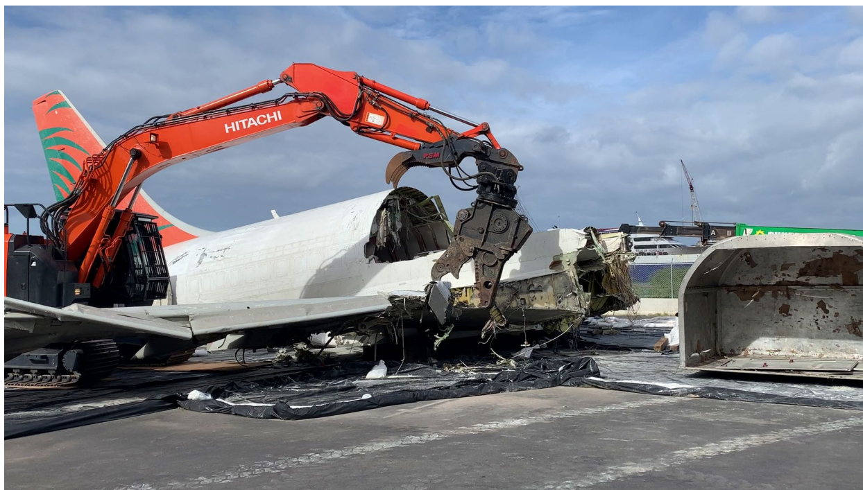
Figure 34. Right wing being cut from the fuselage
