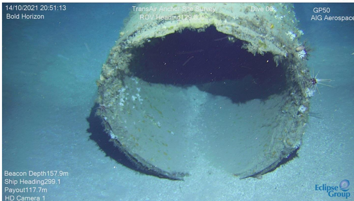
Figure 22. Second view of the same pipe as Figure 21. Appears to be cement. Curious white coral or bryozoan and an urchin on the right side.
