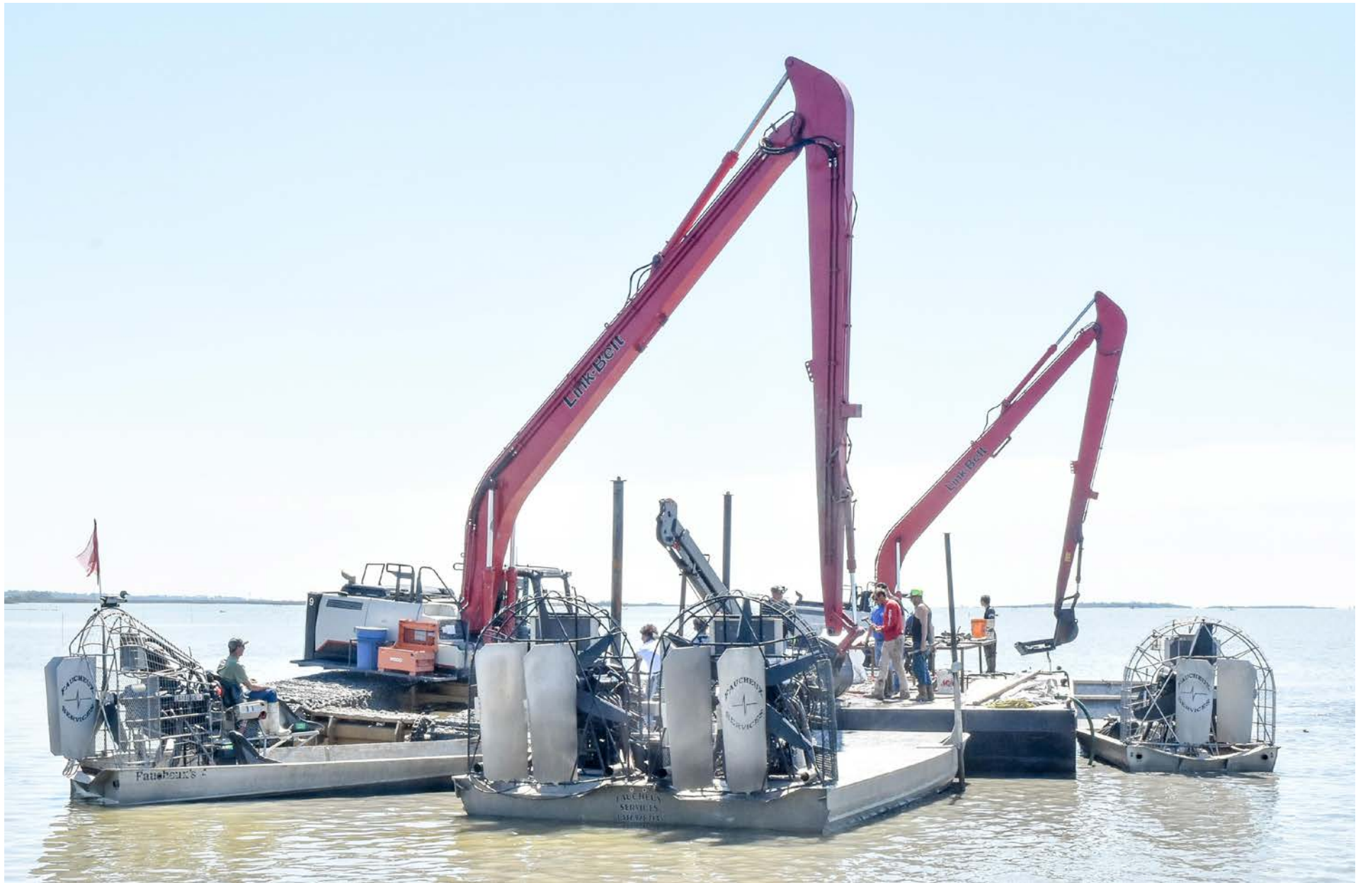
Figure 6 – Shallow water recovery equipment
