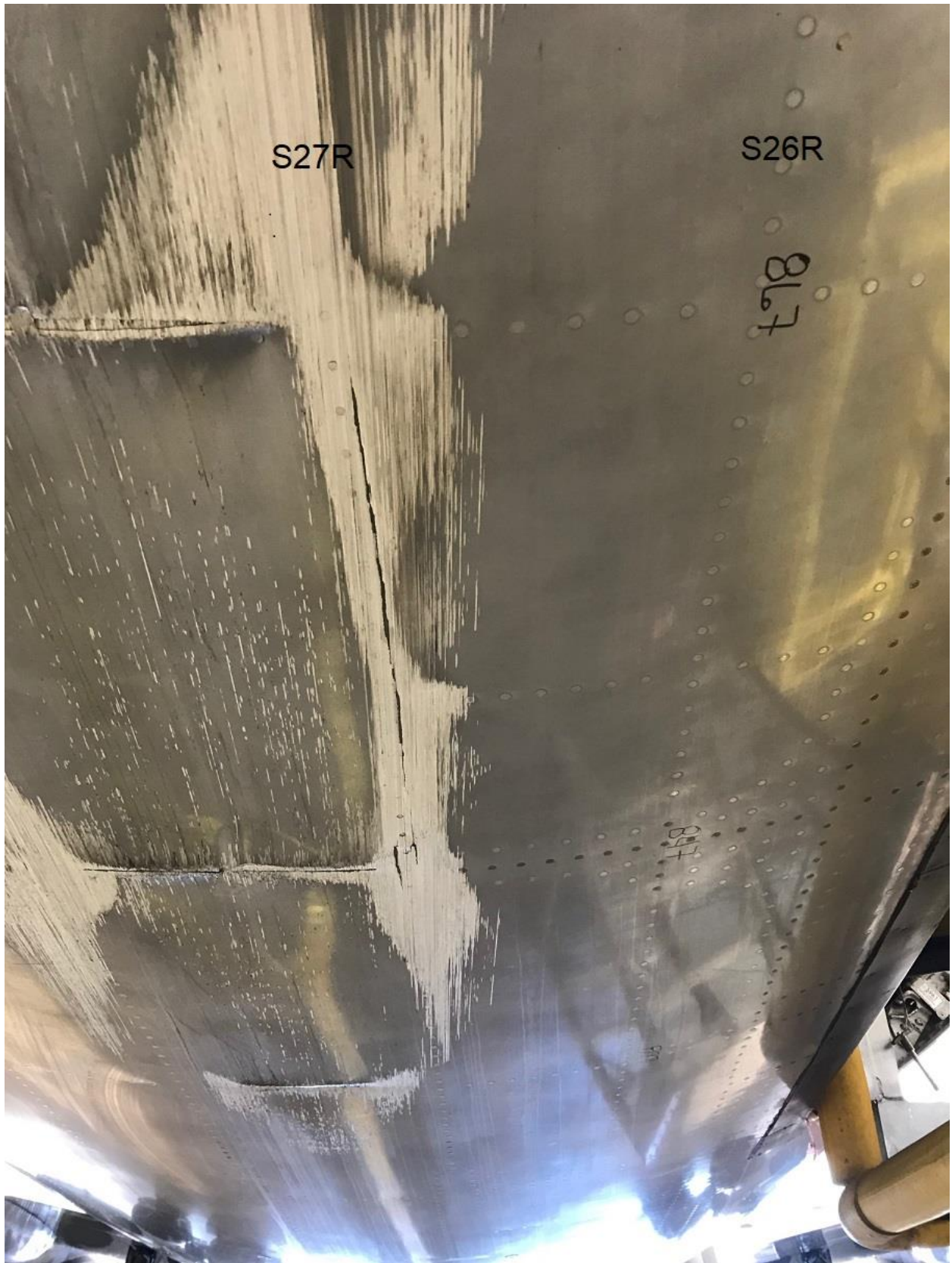
Figure 7 S27 R between STA 847 and STA 867
