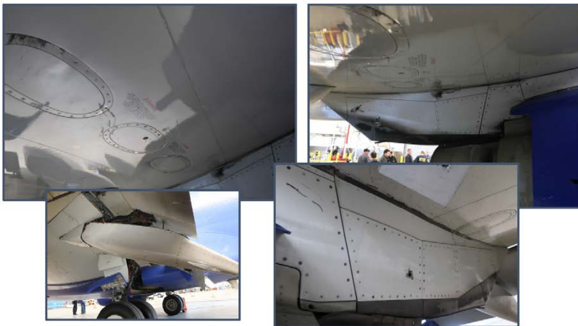
Figure 27 – Wing lower surface damage
