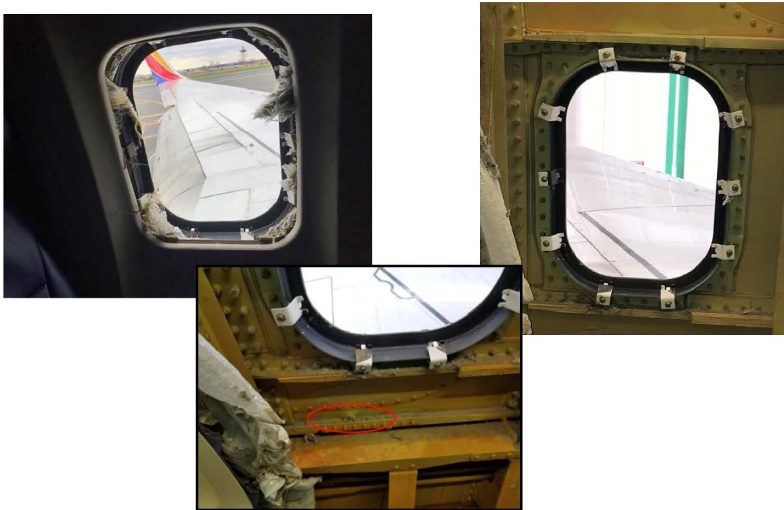
Figure 32 – Interior fuselage impact damage 1
