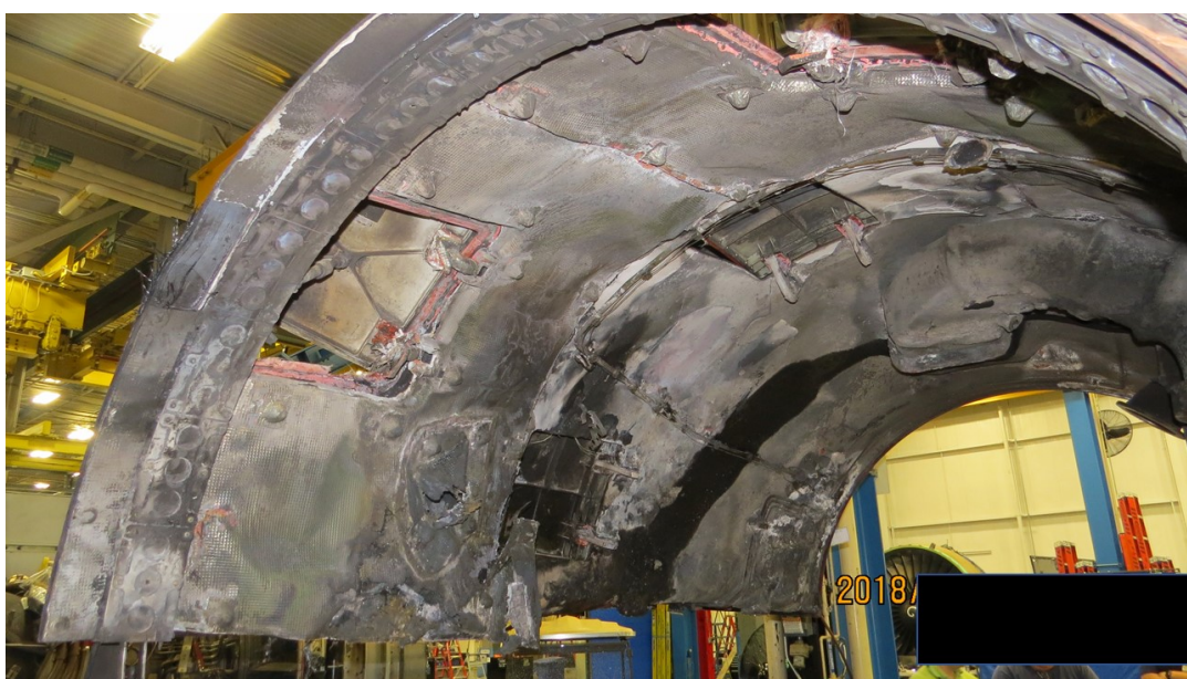
Photo 25- No. 2 Engine Left (Inboard) Thrust Reverser Door IFS Fire Blanket
