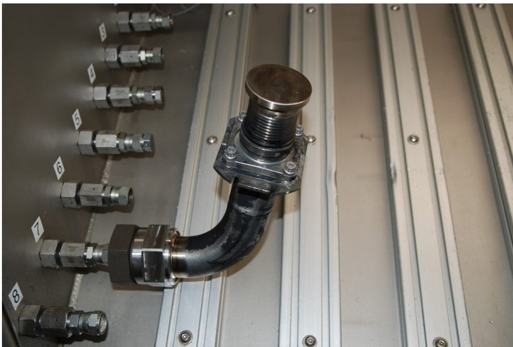
Photo 39- Accident Hardware Installed in Pressure Test Bench
