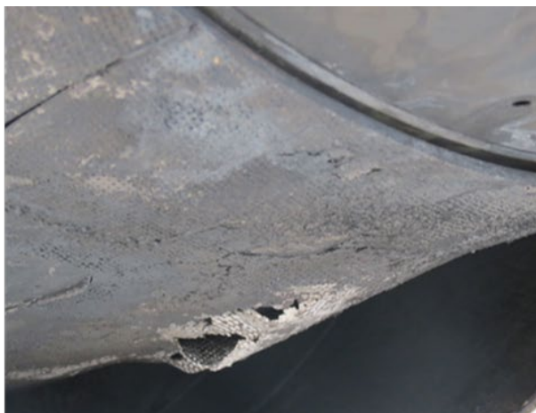
Fig 16. Exposed honeycomb structure in the lower forward core cowl
