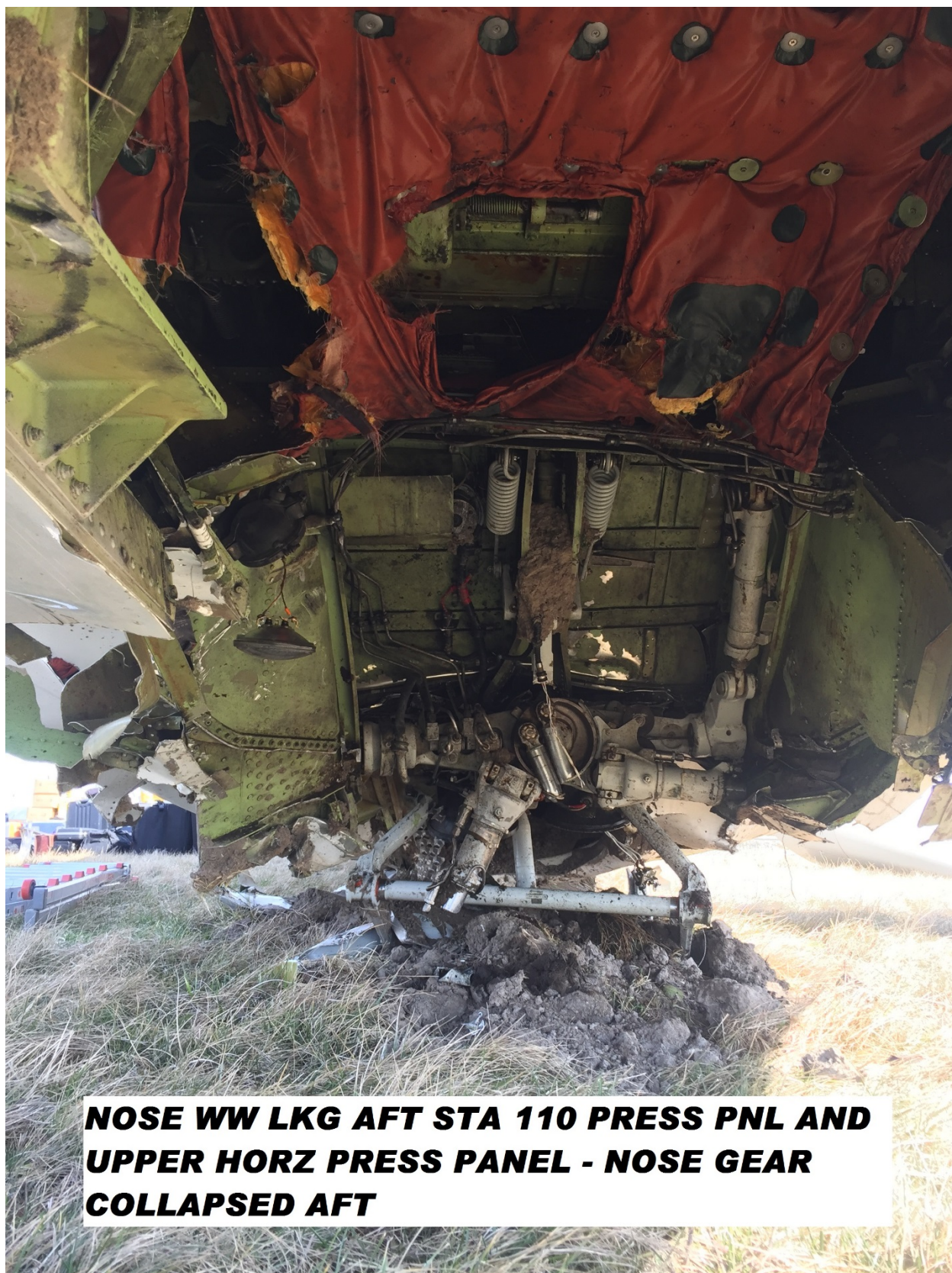
Figure 22 – Nose wheel well damage
