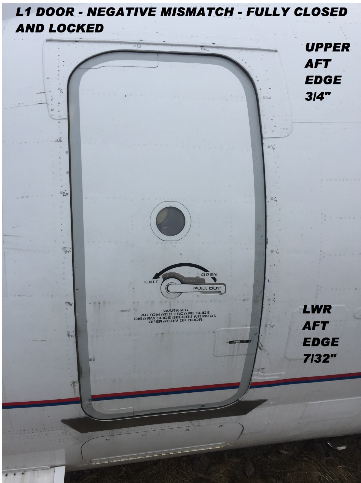
Figure 20 – Main entry door (L1)
