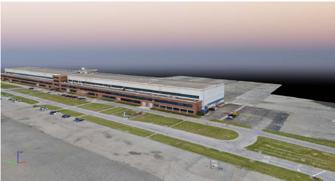
Figure 6 - View of southwestern corner of Hangar 1 at YIP, 3D Model
