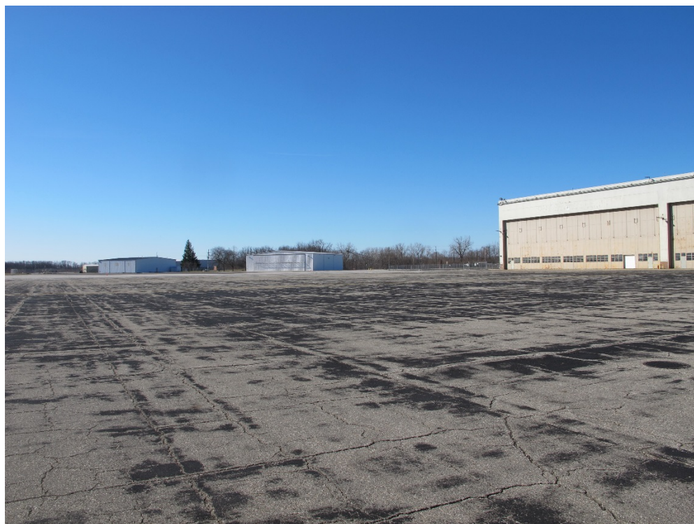
Figure 64 - View looking in a south-westerly direction from approximate aircraft parking location
