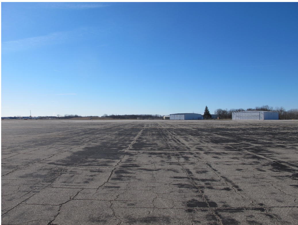
Figure 63 - View looking in a southerly direction from approximate aircraft parking location
