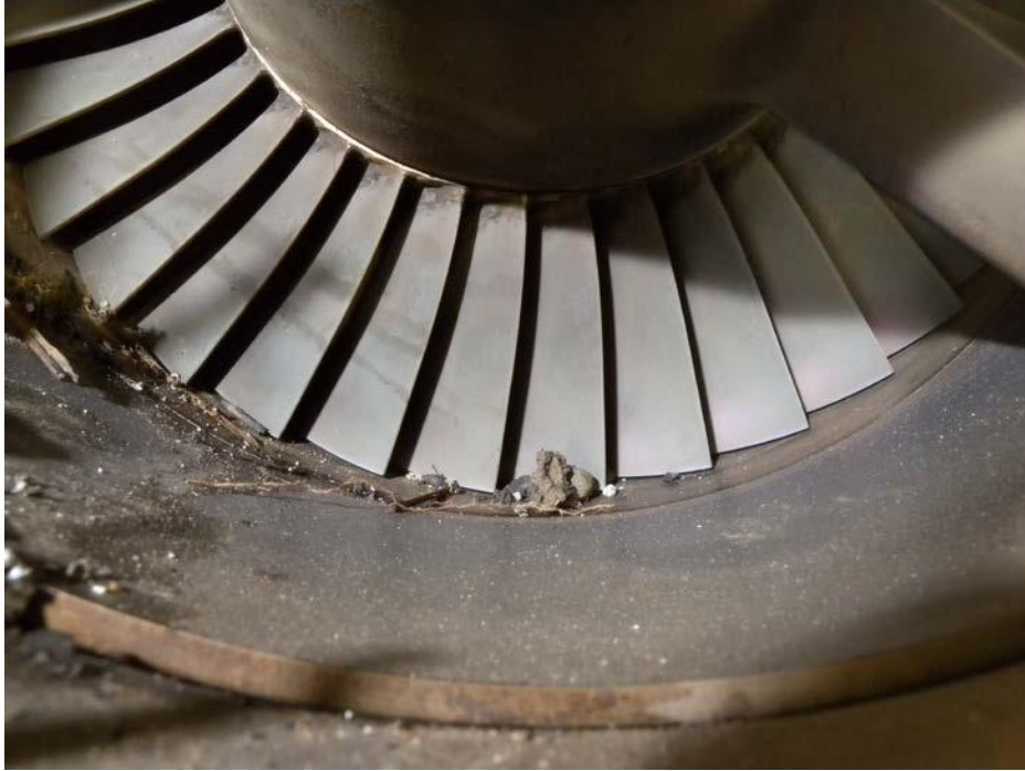
Figure 9 – 3 rd Stage Turbine Wheel – Intact
