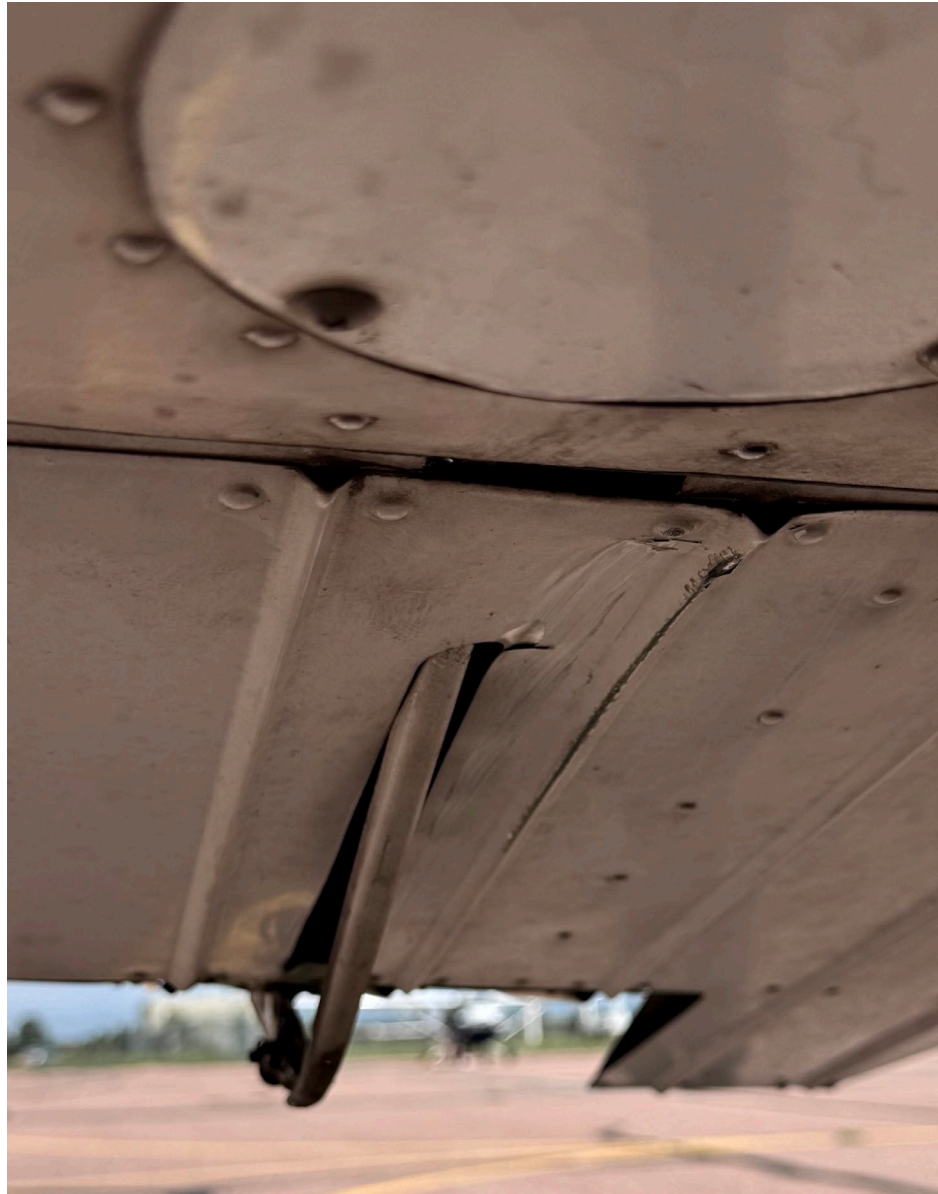
Photograph 4 - Right elevator (Courtesy of USAFA)
