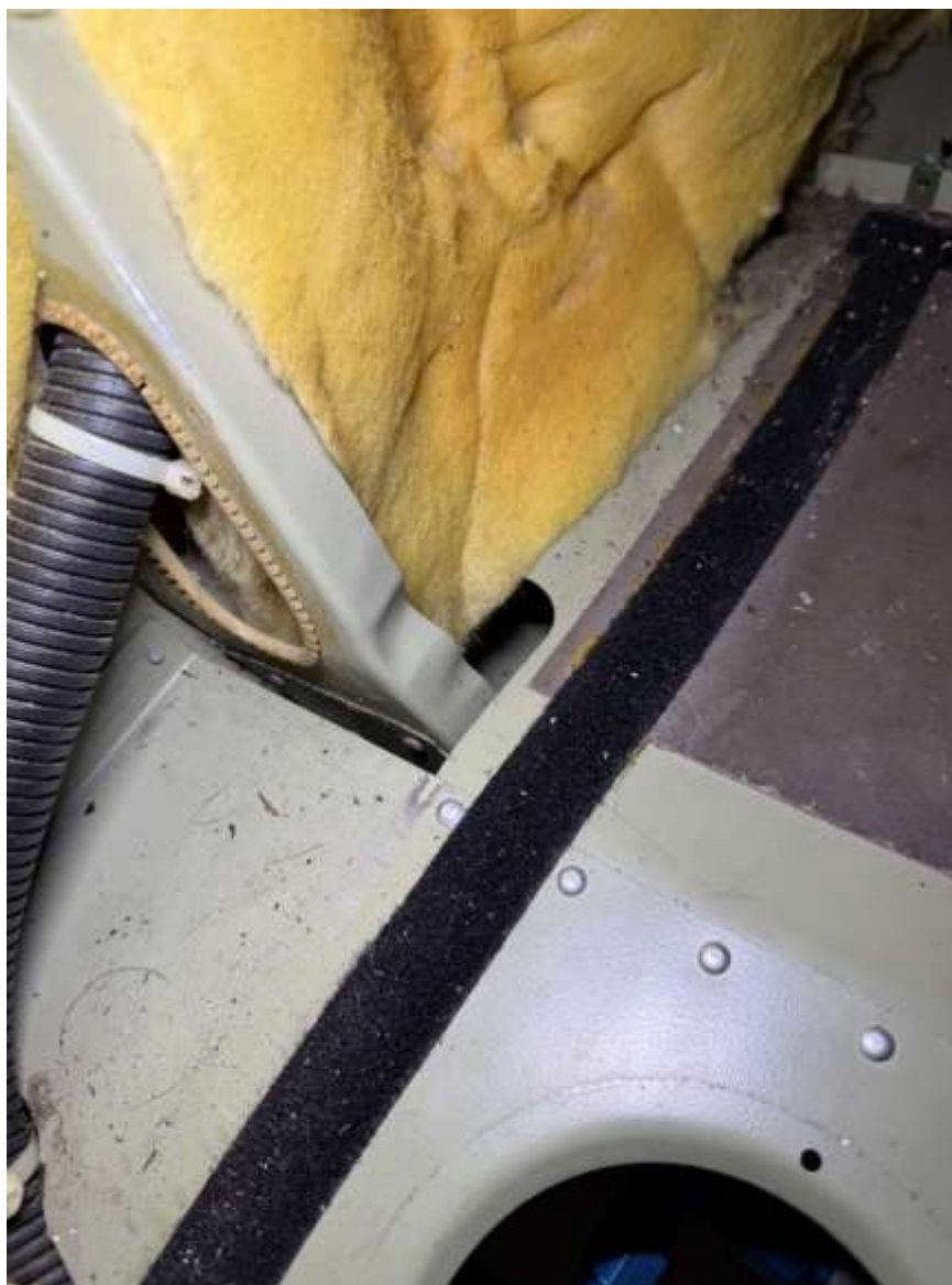
Photograph 1 - Fuselage damage - floor is bowed (Courtesy of pilot)
