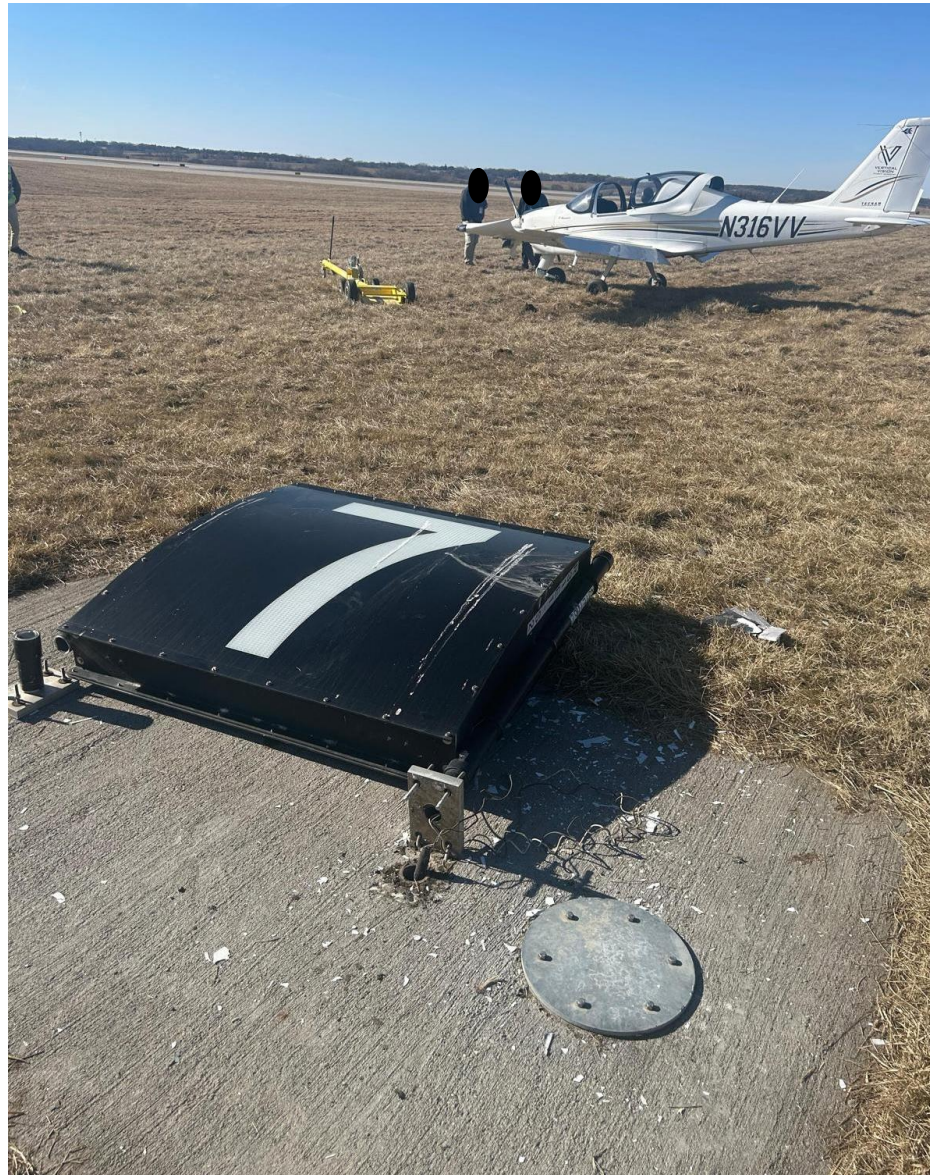
Photograph 2 - Taxiway sign impacted by left wing (Courtesy of flight school)
