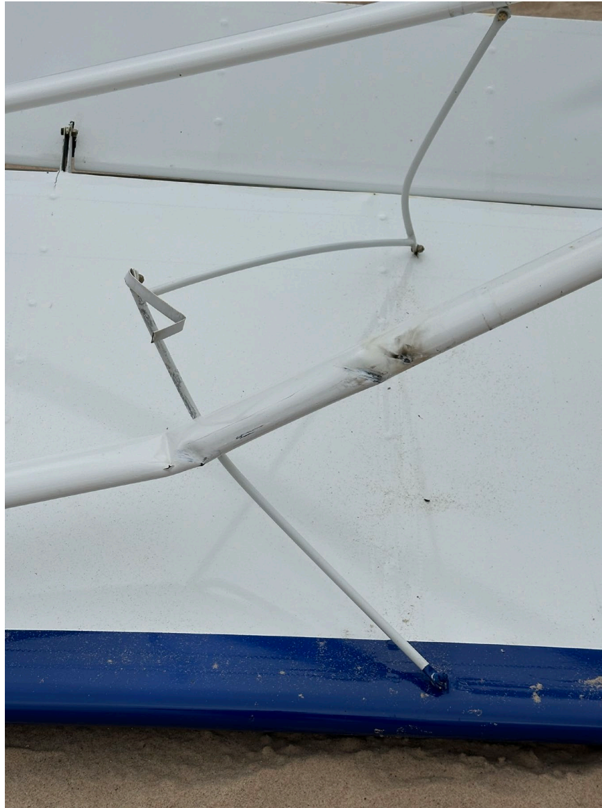
Photograph 4 - Bent wing strut (Courtesy of FAA)
