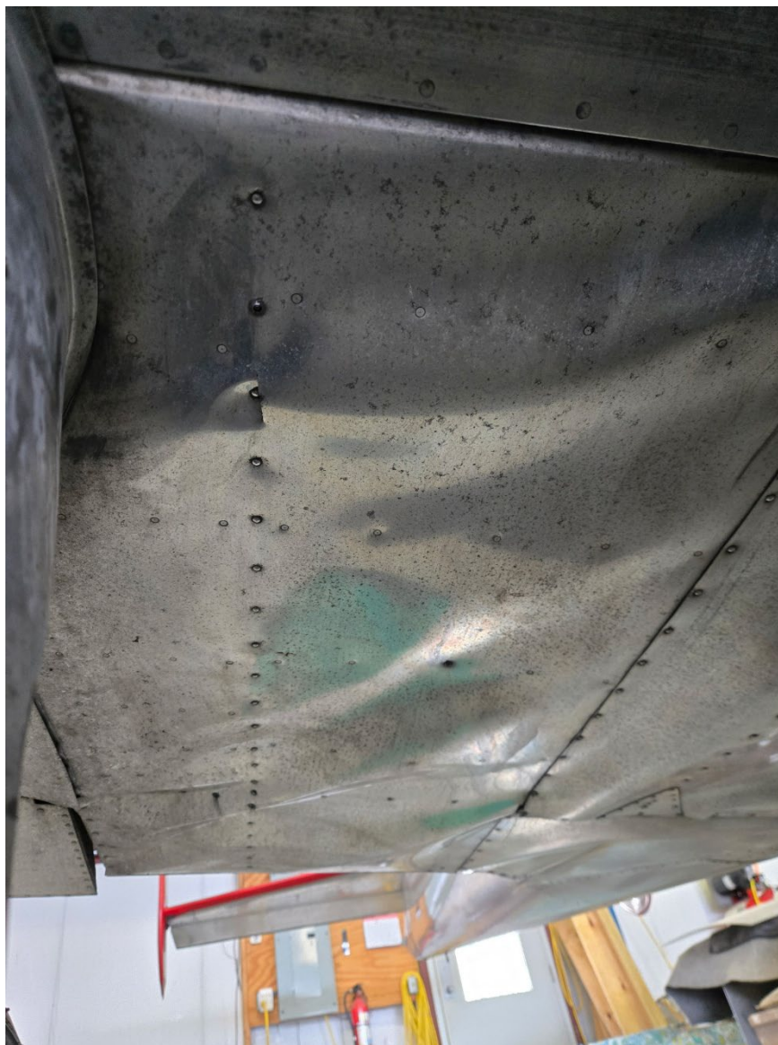
Photograph 2 - Lower Right Wing (Courtesy of Owner)
